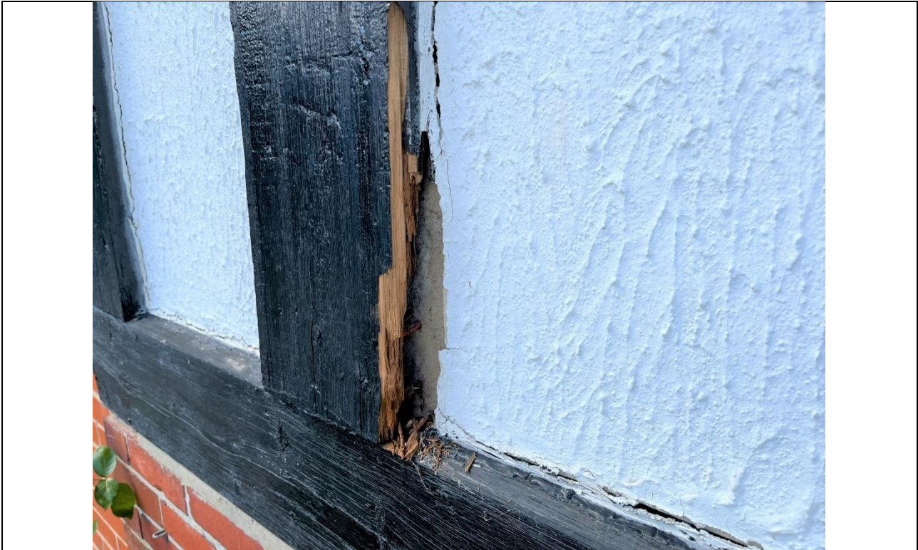
Photo 7 Timber cladding fixed to front wall
