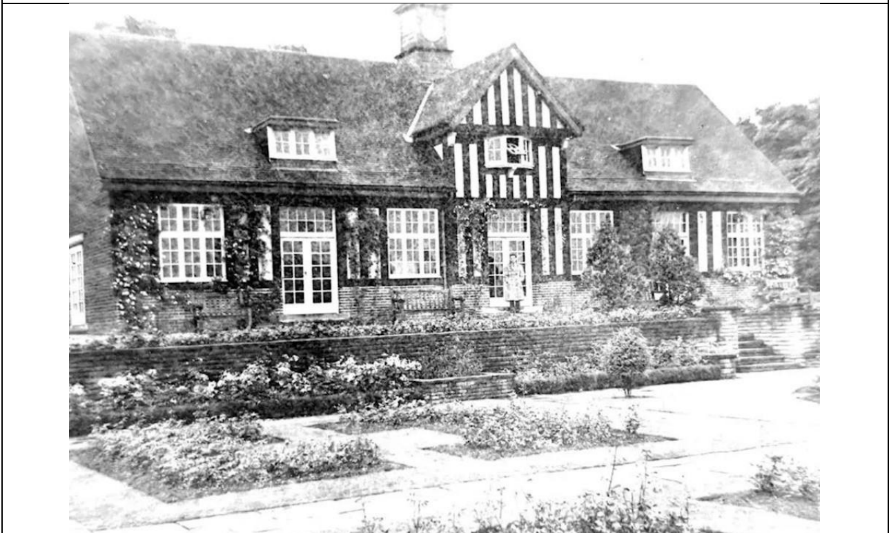
Photo 8 Historic view of the café building
