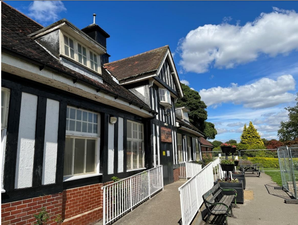
Photo 1 Front elevation looking east
