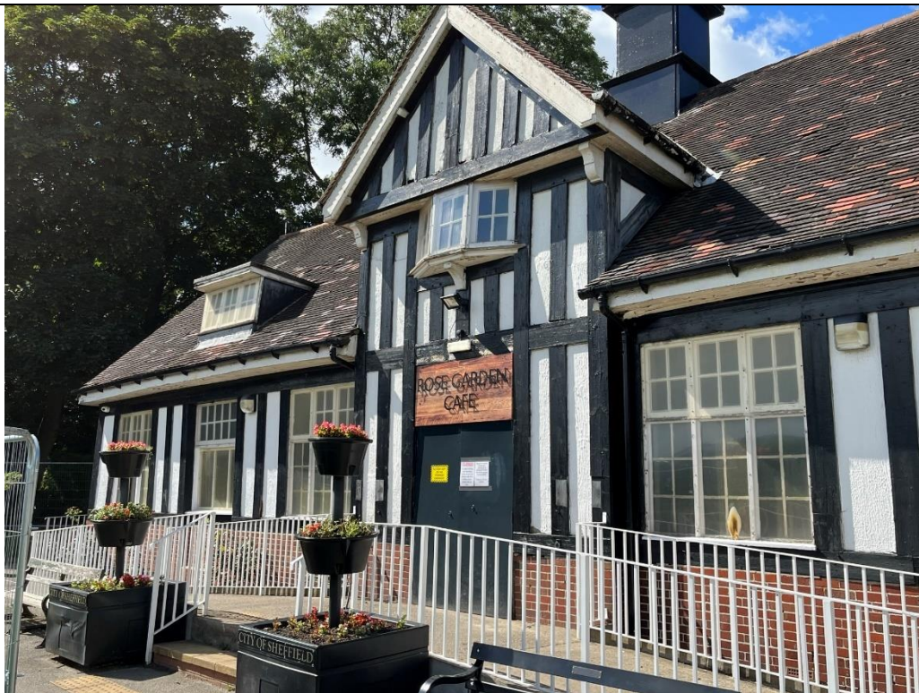
Photo 2 Front elevation looking west
