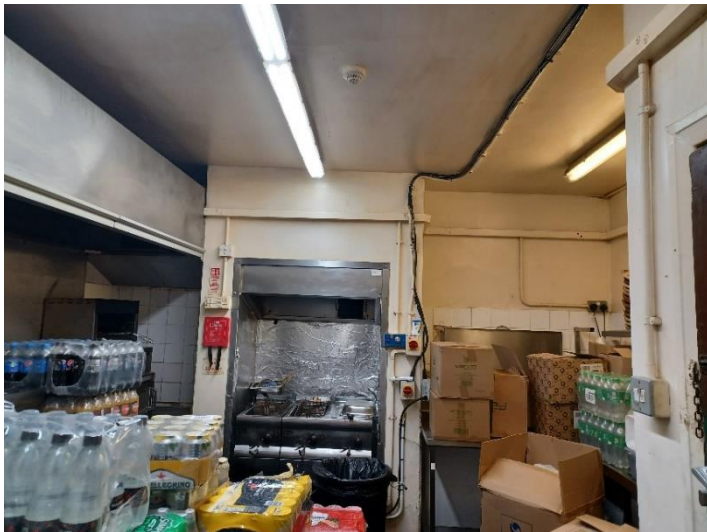
Photo showing existing kitchen facility.
