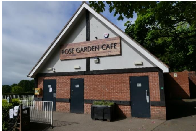
Photo of east facing side elevation of the new WC block to the Rose Garden Café.
