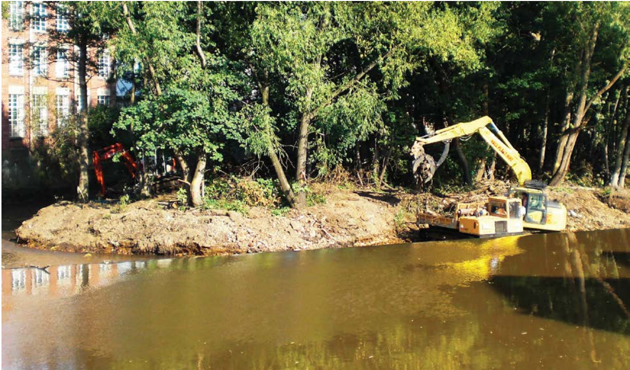
Work by the Environment Agency at Kelham to reduce flood risk by clearing the river channel obstructions. Habitat improvements were made at the same time
