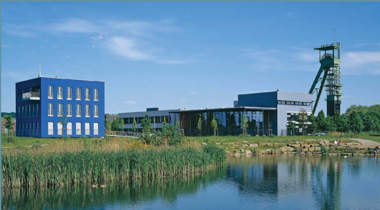
The new landscape and buildings are good but what makes them memorable is the retained pit head gear Photo Credit: LEG GmbH
