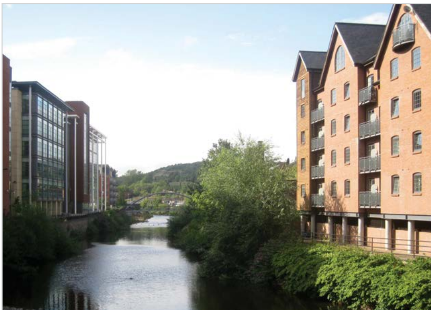
New residential and office development together with a new river walkway in the city centre
