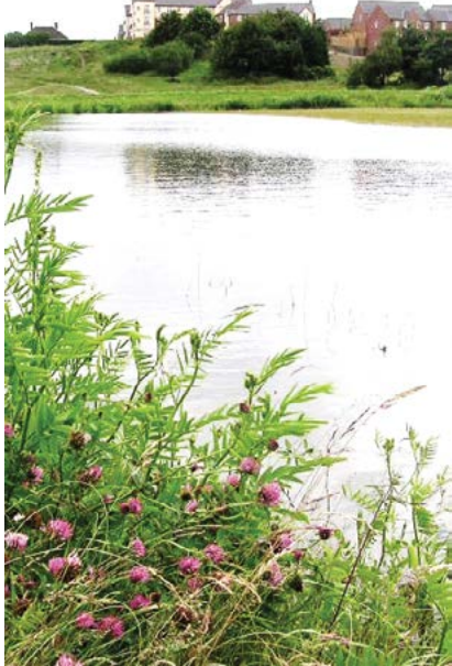
Sustainable drainage. A flood storage basin at the manor holding water after the rainstorm that caused Sheffield's floods in June 2007 Photo Credit: Roger Nowell
