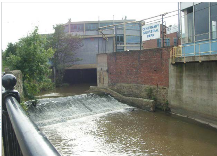
In many places, the rivers have been heavily engineered, this is the Sheaf on Little London Road
