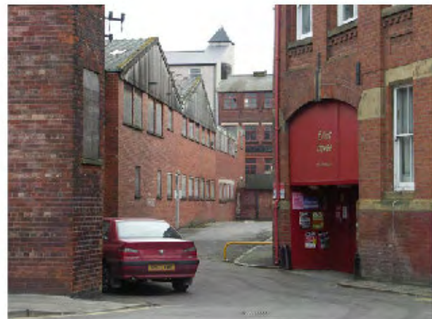
VIEW ALONG SIDE ROAD
